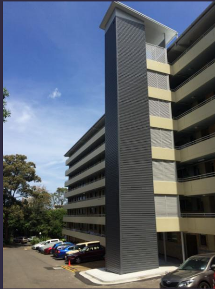
Project Completed at 15 –17 Barton Road, Artarmon
